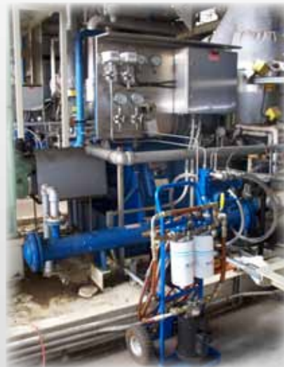
This is the Des-Case filter cart filtering Monolec 6462 in a boiler feed pump. A similar Des-Case filter cart is also used to filter Monolec 6406 in Marley cooling tower gearboxes.
