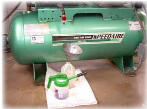
*This Speedair reciprocating compressor is equipped with an Esco Oil Sight Glass. The Oil Safe container holds Monolec 6404 for the compressor.*
