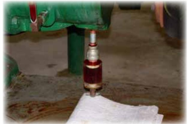
Esco Oil Sight Glasses are installed on these DeLaval pumps.
