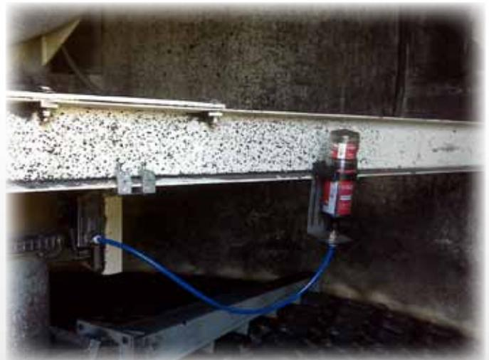
Sometimes the PM was not completed because of time constraints, resulting in equipment not being properly lubricated.
