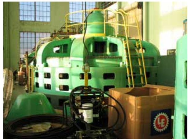
*275-gallon tote and filter cart that was used to transfer the turbine oil into the turbine.*
