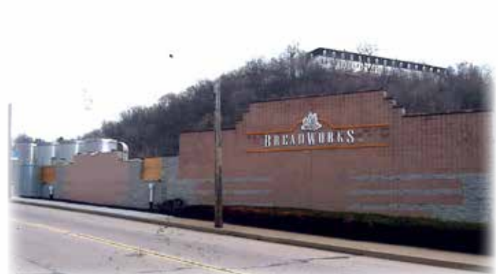
Breadworks Bakery. Note the four flour storage silos on the left. Each silo holds 65,000 lbs of flour.
