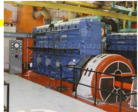
With LE's 8340 MONOLEC PLUS Engine Oil protecting the engine, it did not seize, so the crankshaft required only regrinding and was rechromed, at a cost of only \$35,000. The maintenance personnel were very surprised and very pleased with the performance of LE's 8340. When the crankshaft was installed, the rings were replaced on the original pistons, new liners and bearings were installed, and the unit was returned to service.
