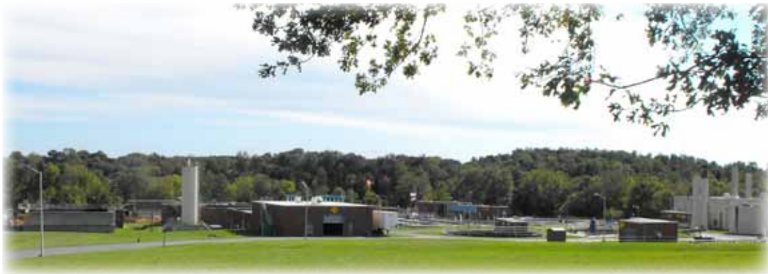
Larger view of the plant
