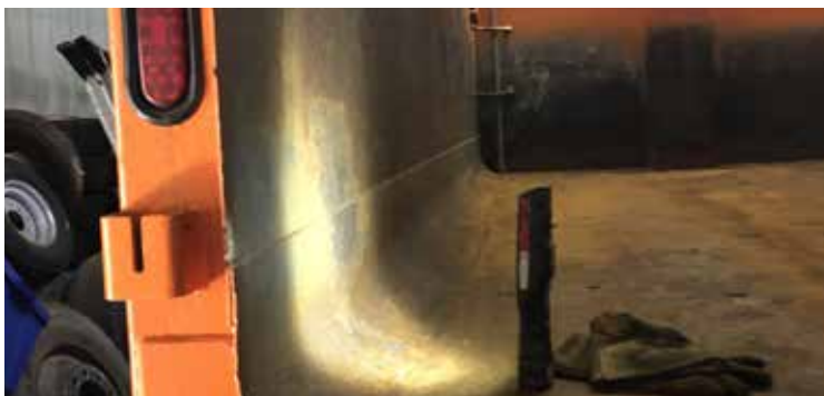
Test patch still rust-free two years after LE's Wirelife Almasol 2002 was applied.
