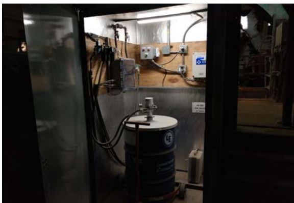
Cement lube room with centralised lubrication system.
