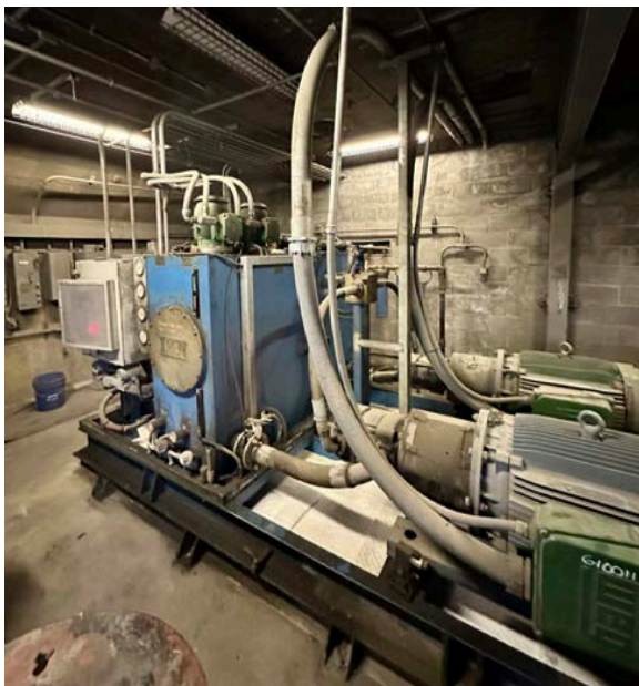
Clinker cooler hydraulic system.
