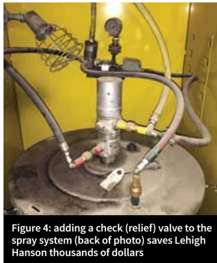
Figure 4: adding a check (relief) valve to the spray system (back of photo) saves Lehigh Hanson thousands of dollars
