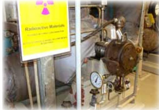
Outboard Heater Drain Pump
