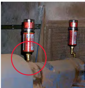
Fan drive shaft lubrication (2 points)
